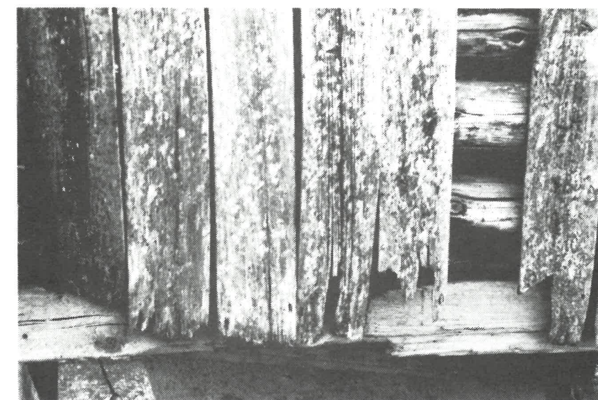
Figure 39: Top, the Chernochan machine shed supported by bracing and standing on timber blocks. Centre, wall logs held together by wooden dowels. Bottom, foundation beam and rotted cladding at the north elevation. (Field Photographs, Chernochan Machine Shed, Sonia Maryn.)
