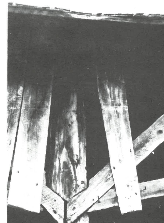
Figure 42: Top, varied wood tone of south elevation (left), and detail showing dowel pegging. Bottom, log wall to post connection at northeast corner (left) - note wedge closing gap between logs, and central post of east elevation - note notching at knee brace. (Field Photographs, Chernochan Machine Shed, Sonia Maryn.)
