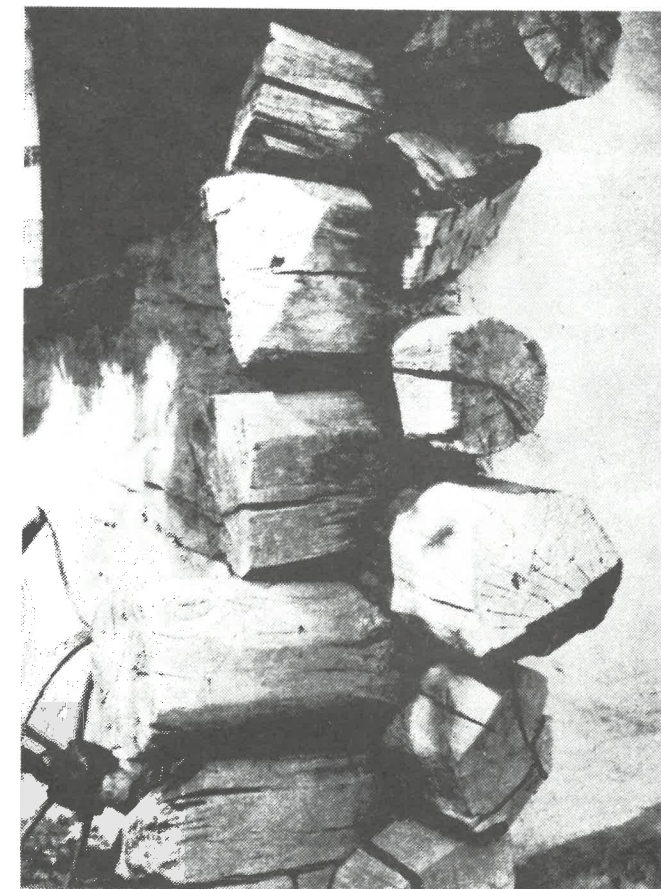
Figure 40: Top, notching at the southwest corner, interior (left) and exterior views. Bottom, the exterior of an untrimmed saddle-notched corner in Ukrainian house. (Field Photographs, Chernochan Machine Shed, Sonia Maryn and Figure 22 in Z.S. Hudchenko, Muzei . Kiev: Budivelnik, 1981.)
