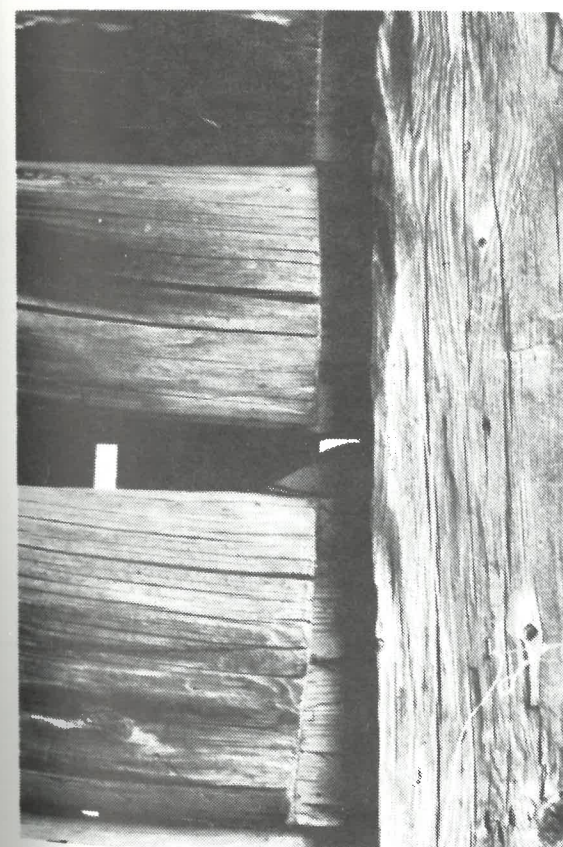
Figure 42: Top, varied wood tone of south elevation (left), and detail showing dowel pegging. Bottom, log wall to post connection at northeast corner (left) - note wedge closing gap between logs, and central post of east elevation - note notching at knee brace. (Field Photographs, Chernochan Machine Shed, Sonia Maryn.)
