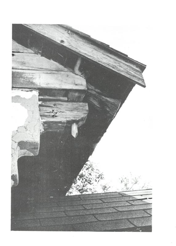
Figure 7. Roof pegging at eave. Stepped eave bracket at left.
