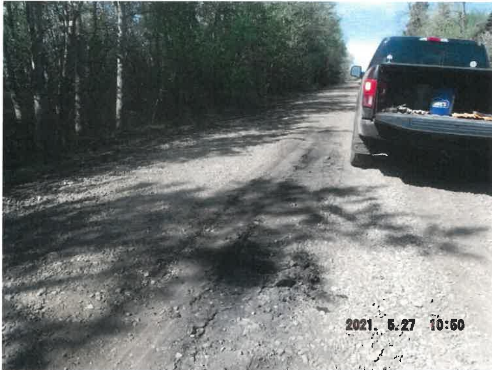
Photograph 13: Looking at the ruts within Alignment 6
