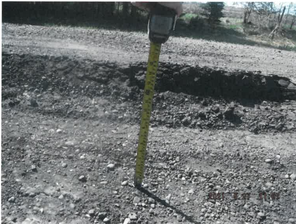
Photograph 11: Looking at ruts within Alignment 5
