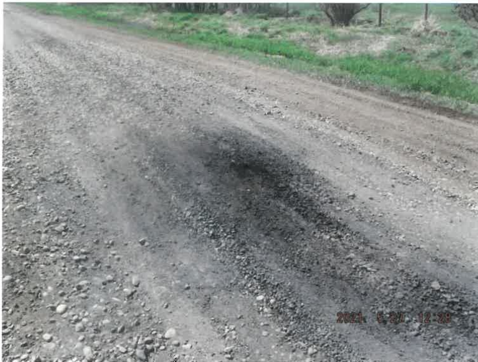
Photograph 3: Looking at exposed organic soil within Alignment 1
